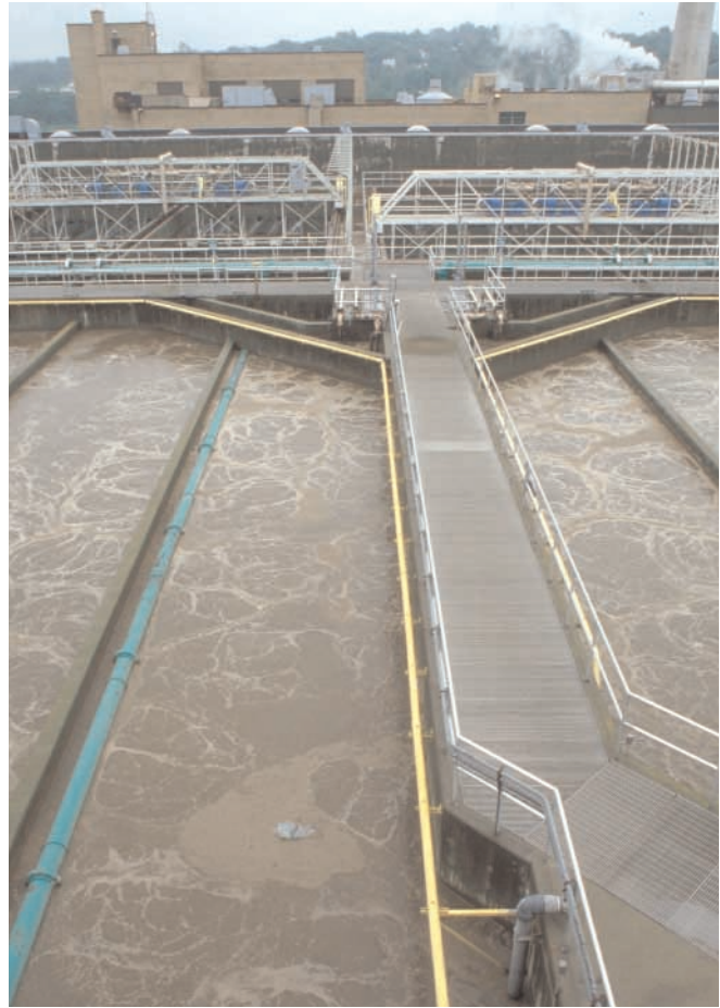
Water treatment often involves a large geographic area, requiring remote automation sites.
